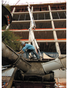
A worker oversees a final concrete pour for the RRF.
