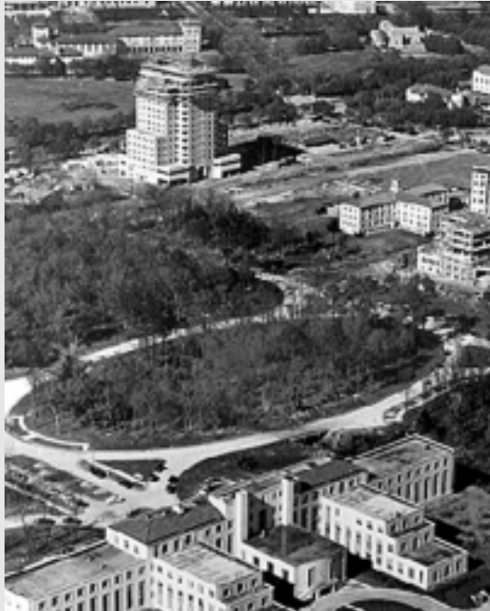
The Hermann Professional Building, upper left, under construction in the summer of 1948.
