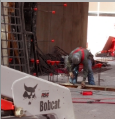
Completion of the hydrostatic wall is a top priority.
